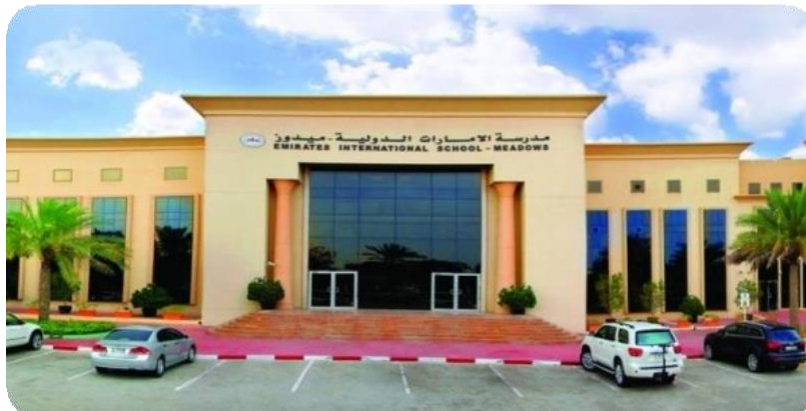
Emirates International School Expansion - Dubai
