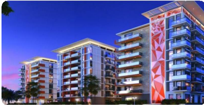
Celestia – Luxury 950 Rooms Hotel Apartment, Dubai South
