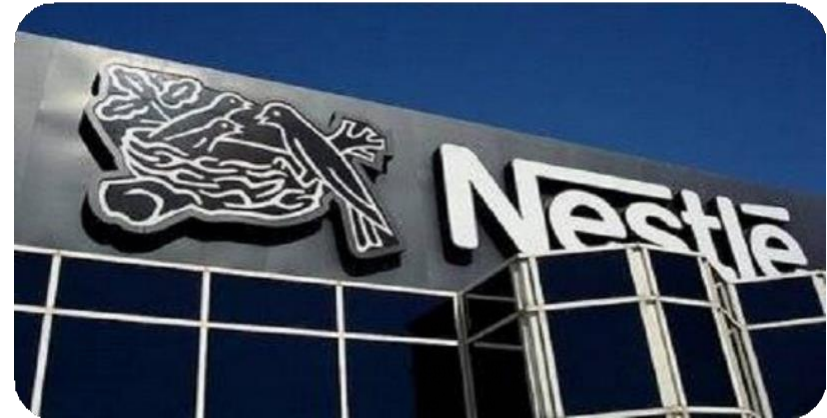
Nestle Manufacturing Plant Dubai World Central (DWC)
