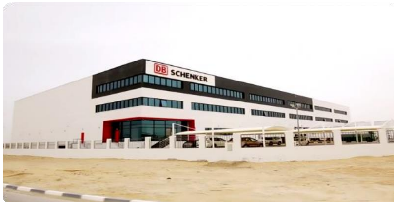
DB Schenker Office & Warehouse, DWC
